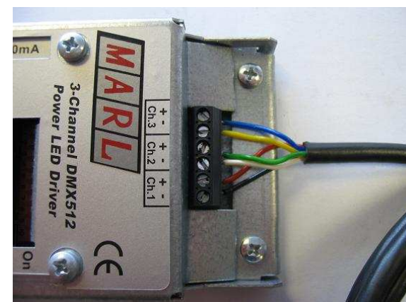
WIRING OF FIXTURE
